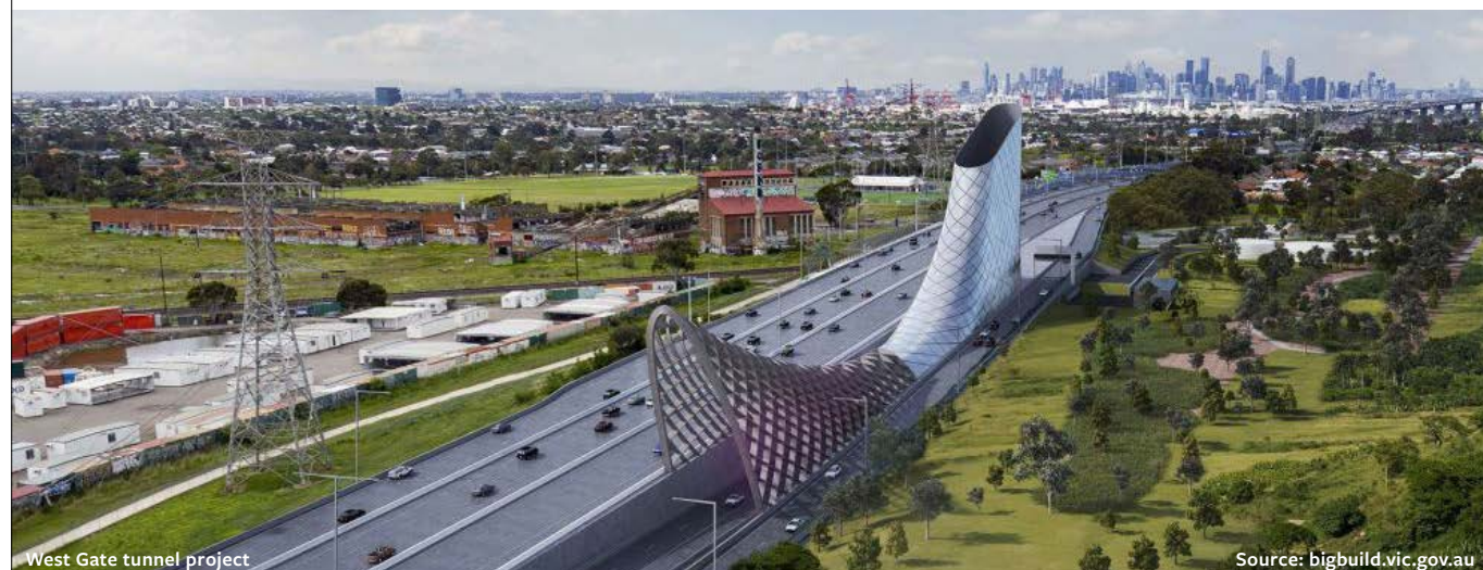
West Gate tunnel project
