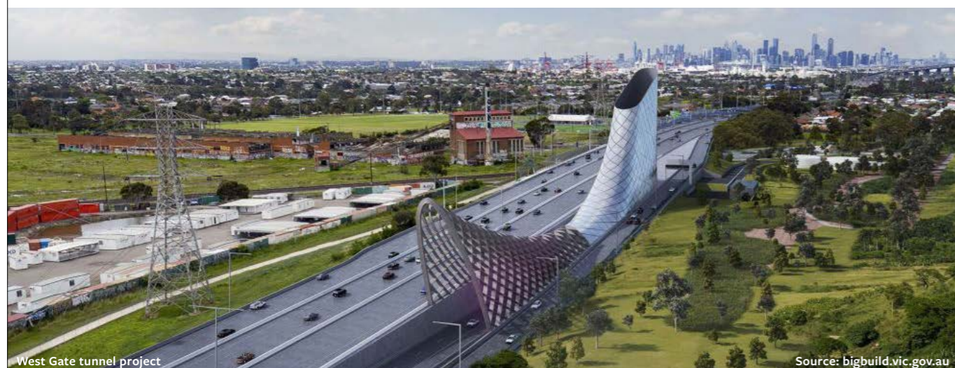
West Gate tunnel project
